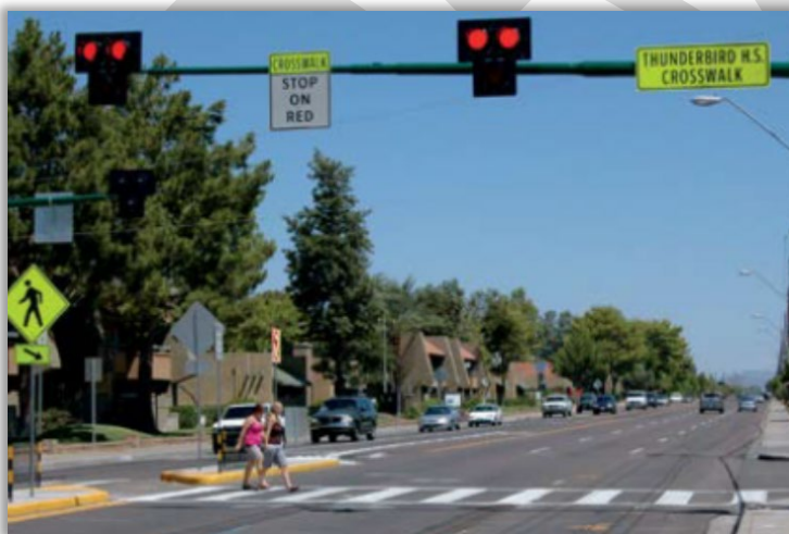
Figure 62: Pedestrian Hybrid Beacon (PHB)
